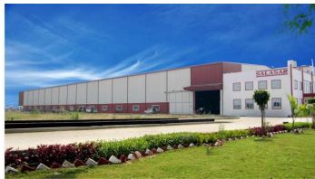
Salasar Techno Engineering's new galvanising plant to begin functioning early-next year: MD
